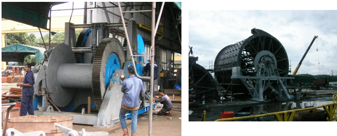
Figure 1a and 1b: Work at Plimsoll Corp Pte Ltd
